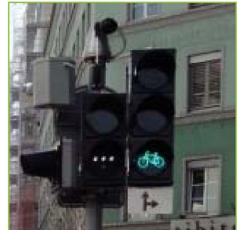
The traffic light is equipped with a camera that detects approaching cyclists. An object is defined as ‘cyclist’ if it moves through certain fields but not others (see picture below).
